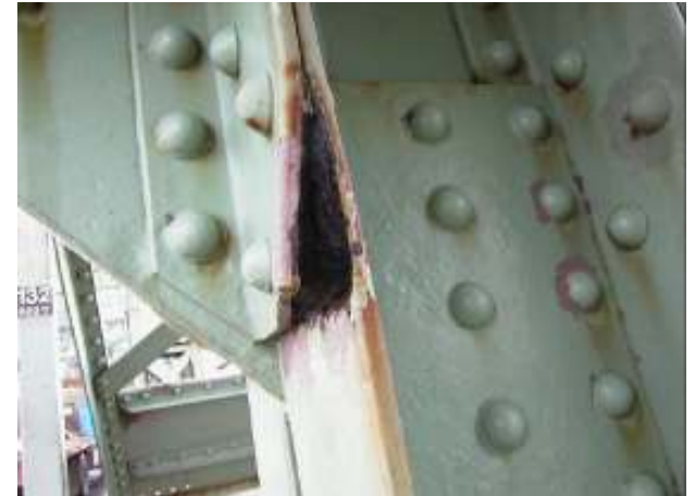
Crevice corrosion
